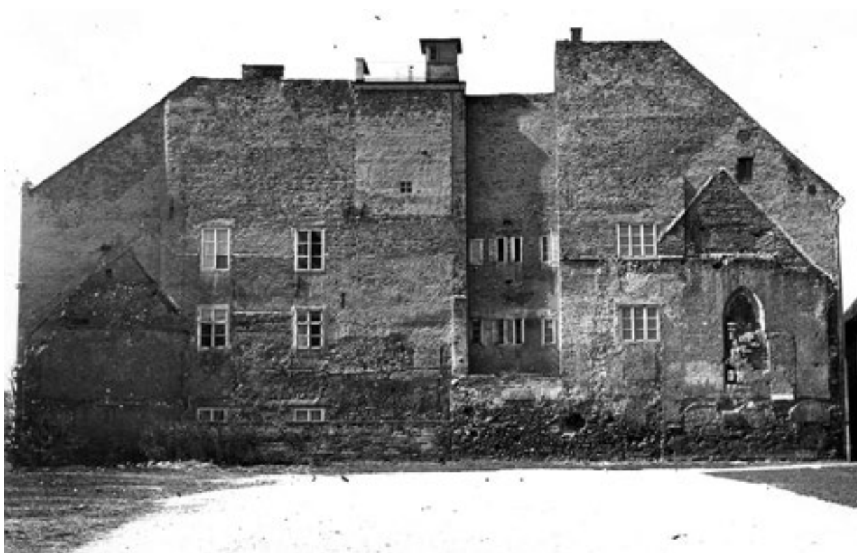
4. Istočni zid zgrade Hidrometeorološkog i Geofizičkog zavoda s obrisom kapucinske crkve, očuvanim gotičkim prozorom i kompozicijom spolija unutar prozora (desno) te obris bivšeg kapucinskog samostana (lijevo) (fototeka MGZ-a, 10422 a, snimio J. Vranić, 1972.) East wall of the Meteorological and Hydrological Service building with the outline of the Capuchin church, a preserved Gothic window and a composition of spolia inside it (right) and the outline of the former Capuchin monastery (left) (Zagreb City Museum Photo Archive 10422 a, photo by J. Vranić, 1972)
