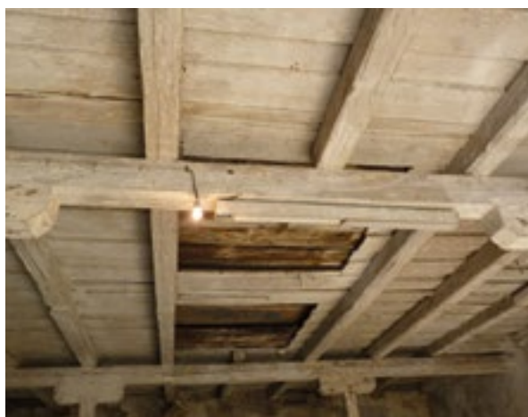
16. Drveni strop konjušnice s nekadašnjim otvorima za odračivanje (fototeka HRZ-a, snimila I. Pauk Sili) Wooden ceiling of the stables with former ventilation openings (Croatian Conservation Institute Photo Archive, photo by I. Pauk Sili)
