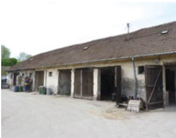
3. Pogled na istočno pročelje velike Hornwerk vojarne (fototeka HRZ-a, snimila I. Pauk Sili) View of the east front of the Large Hornwerk Barrack (Croatian Conservation Institute Photo Archive, photo by I. Pauk Sili)
