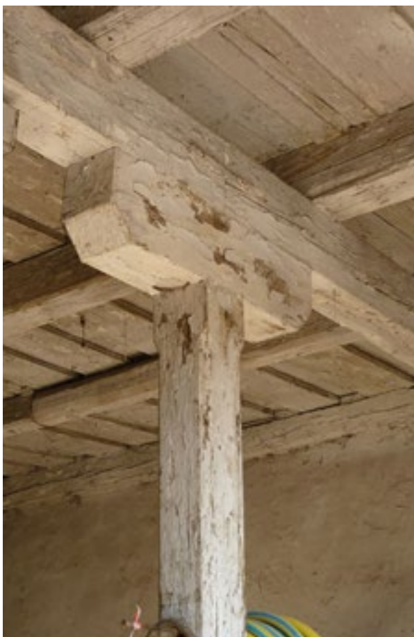
14. Drvena konstrukcija – nosiva greda, vuta i stup (fototeka HRZ-a, snimila I. Pauk Sili) Wooden construction: support beam, haunch and column (Croatian Conservation Institute Photo Archive, photo by I. Pauk Sili)
