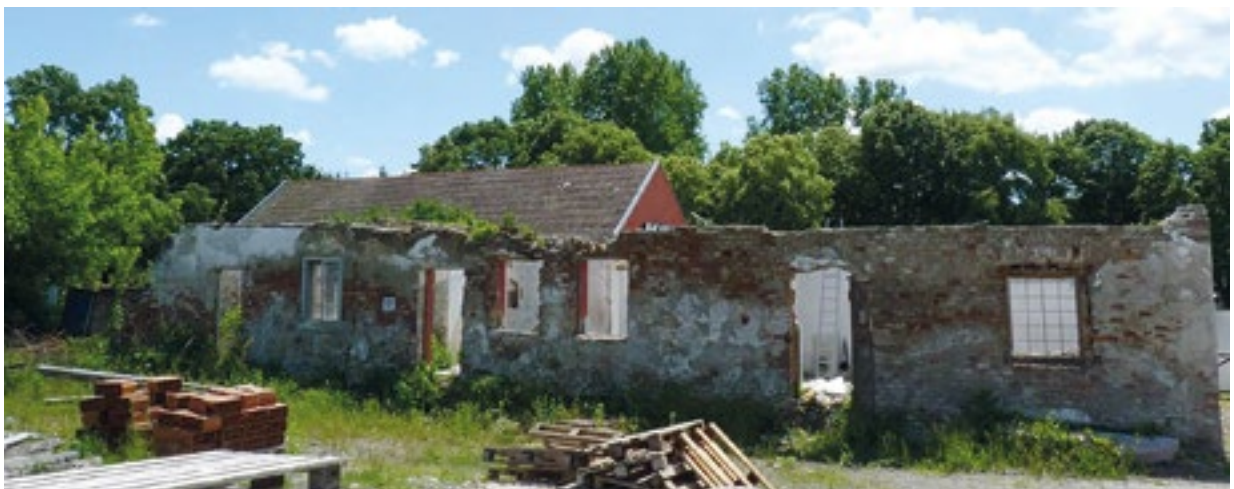
2. Pogled na sjeverno pročelje zatečenog ostatka male Hornwerk vojarne (fototeka HRZ-a, snimila I. Pauk Sili) View of the north front of the Large Hornwerk Barrack remains (Croatian Conservation Institute Photo Archive, photo by I. Pauk Sili)
